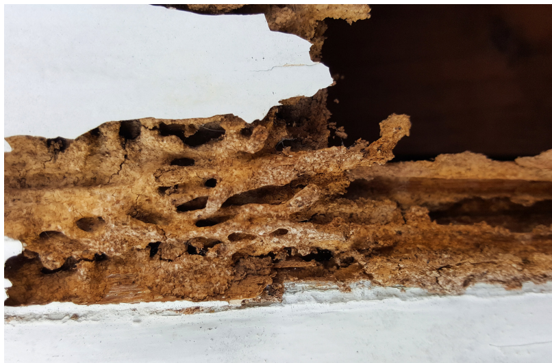
Signs of termite damage: mud “tubes” on foundation surfaces and hollowed wood.
