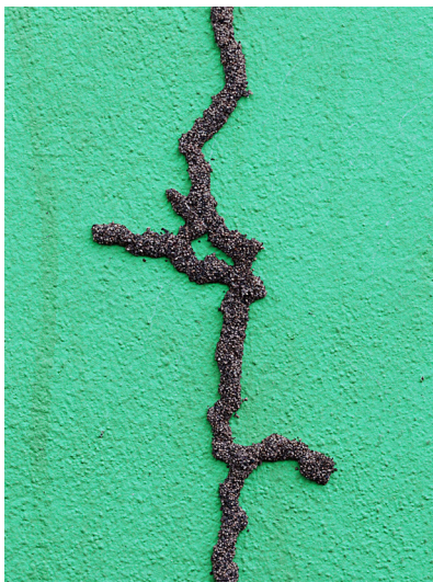
Signs of termite damage: mud “tubes” on foundation surfaces and hollowed wood.
